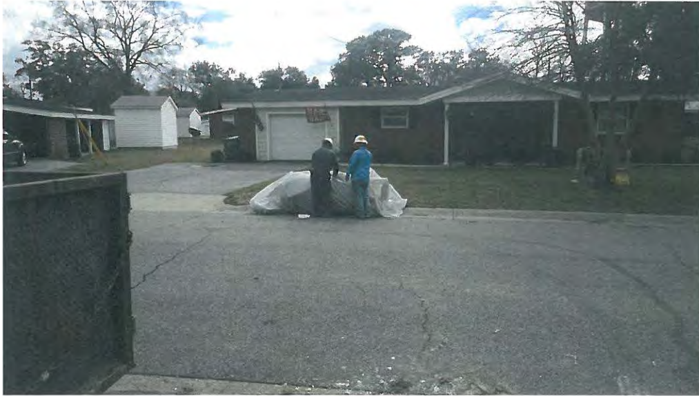
Picture 3: UST 563Dahlia being wrapped for transport.
